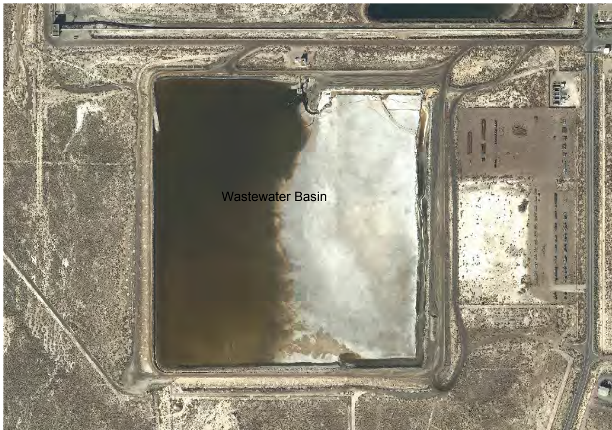
Figure 3-1 – Wastewater Basin Current Conditions
